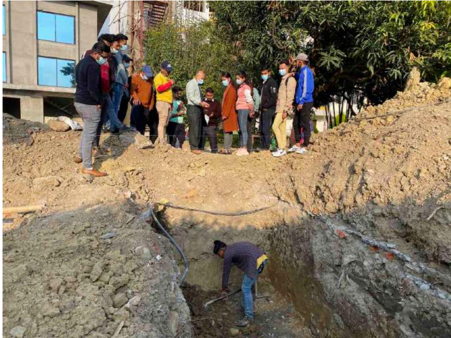
5.2 Field Visit (Observing Construction Site)
